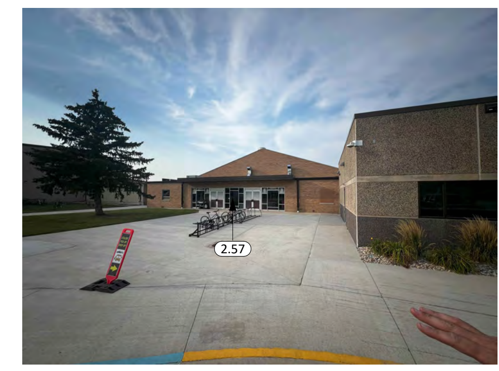
EXISTING PHOTO Z • ALTERNATE #3, REMOVE STOREFRONT FRAMING
